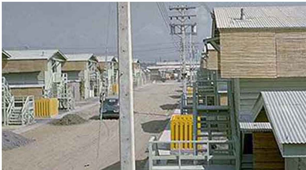
SPS barracks in Dec 1967.
