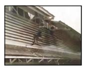
Pictures of damaged hooch. Round blew through the roof, Glanced off the side, detonated & fragged the whole wall
