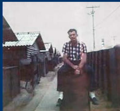
6) Turner sitting on top of a small revetment wall designed to contain flying shrapnel from mortars or rockets.
