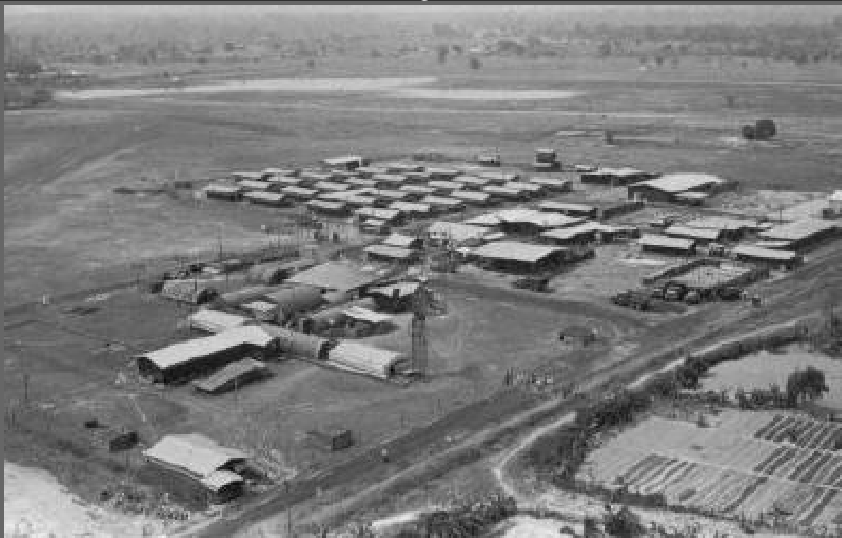
Mukdahan - Fly over: Radar, center photo.
