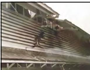
Pictures of damaged hooch. Round blew through the roof, Glanced off the side, detonated & fraged the whole wall
