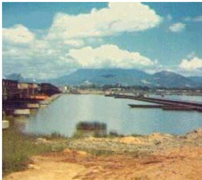
[2] Temporary pontoon bridge to right. Bridge to left was blown.
