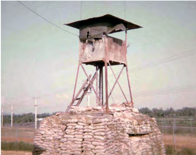
29. Da Nang AB, East perimeter SP Tower.
