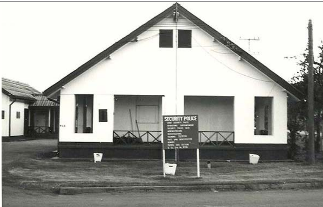
5. Don Muang AB, 631st SPS, CSC building.
