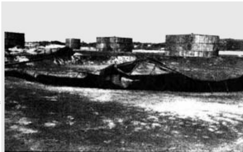
This is the remains of the POL tank involved in the Sapper attack. refer to the story 'Smelling like a Rose' The tanks in the back ground showed effects of the intense heat but did not burn, they were filled with JP4 We were lucky that other tanks did not explode causing more damage. There were satchel charges placed at other tanks but they did not cause the fire this one did
