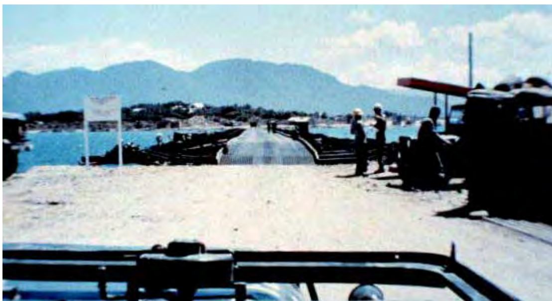
15) Floating Bridge at CRB.
