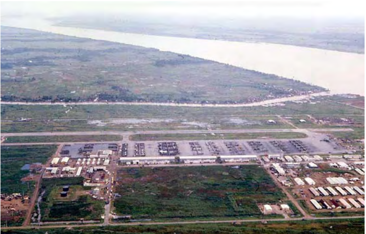
21. Binh Thuy Air Base, flight line view. Mekong Delta-6 tower, West view. MSgt Summerfield.
