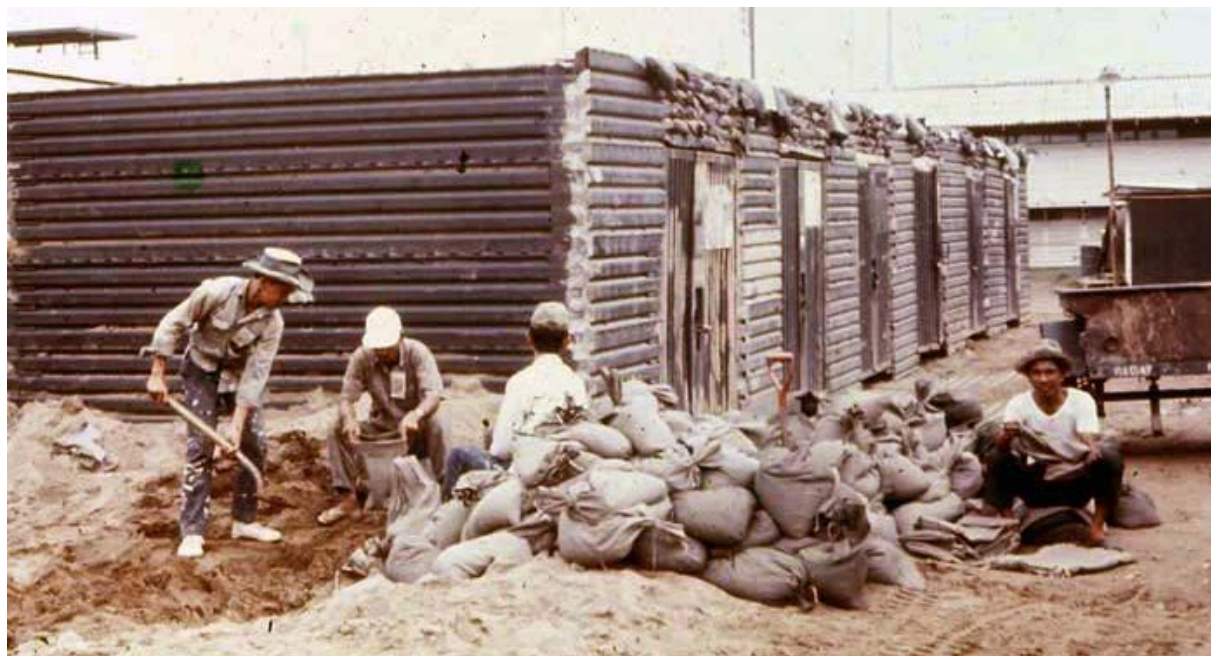
Binh Thuy Air Base, Vietnamese workers are either sandbagging , or filling sandbags, during bunker construction next to ammo storage revetments. MSgt Summerfield: 33
