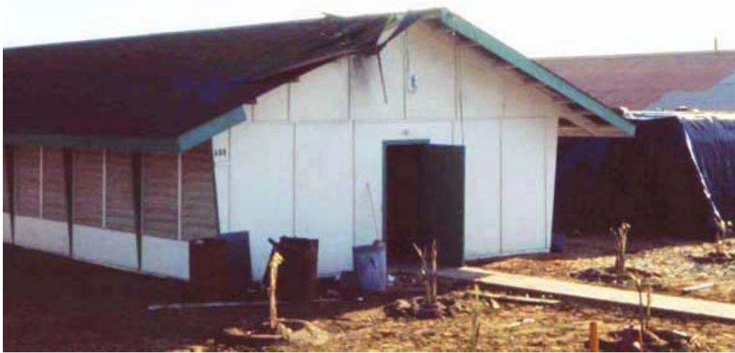
Binh Thuy Air Base, rocket damage. MSgt Summerfield, 1968: 38
