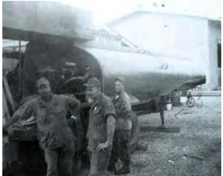
8. Firemen by a larger converted fuel tanker for foaming the runway faster.
