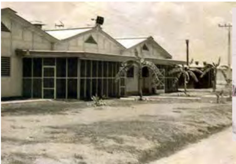
23. The new modern chow hall at Binh-Thuy.
