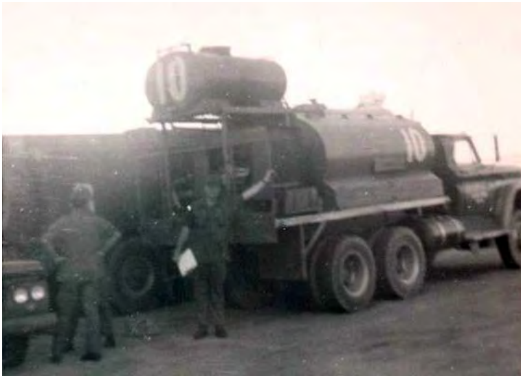
7. We modified a water tanker truck so it could foam the runway.
