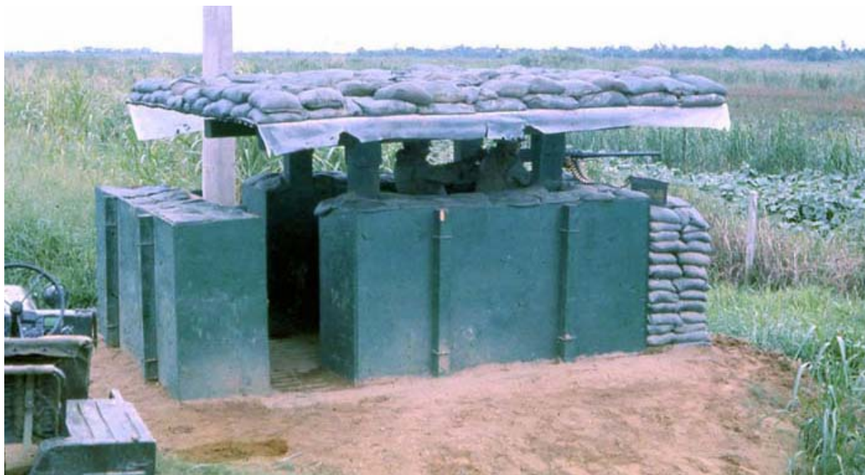
Binh Thuy Airbase, SPS Airman mans perimeter-bunker with 50cal. MSgt Summerfield: 06
