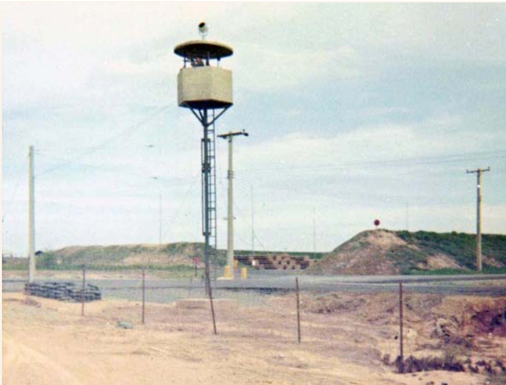
2a. Bien Hoa AB, Ammo Dump Tower. Photo by Ernest Govea, BH, 3rd SPS, 1966-1967.
