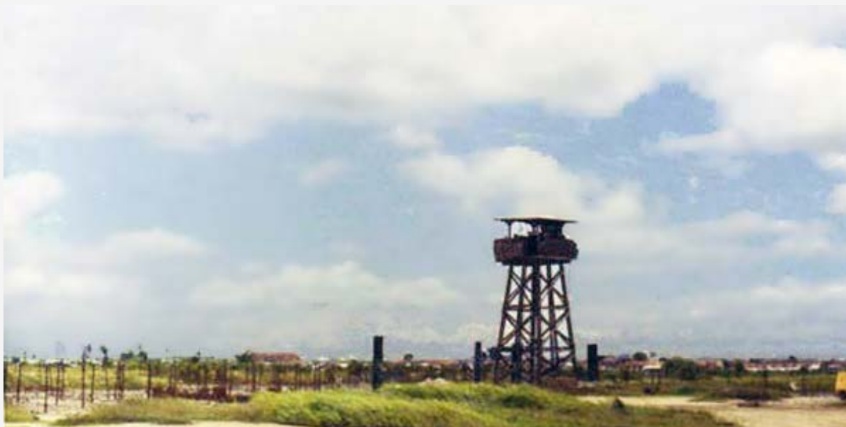
4. Bien Hoa AB, Perimeter Tower. Photo by Ernest Govea, BH, 3rd SPS, 1966-1967.
