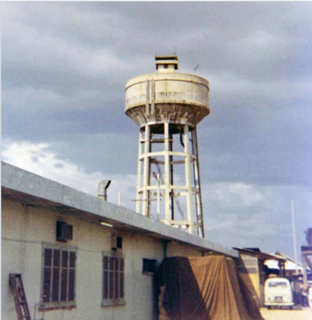
5. Bien Hoa AB, Water Tower. Photo by Ernest Govea, BH, 3rd SPS, 1966-1967.
