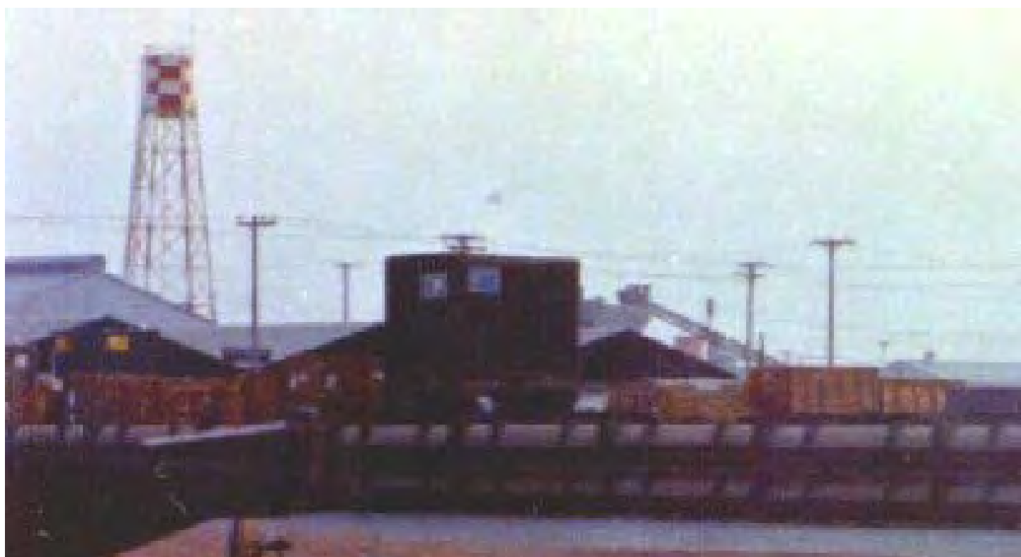
31. Water Tower visible from most of Bien Hoa AB, and prominent from the SPS Compound.
