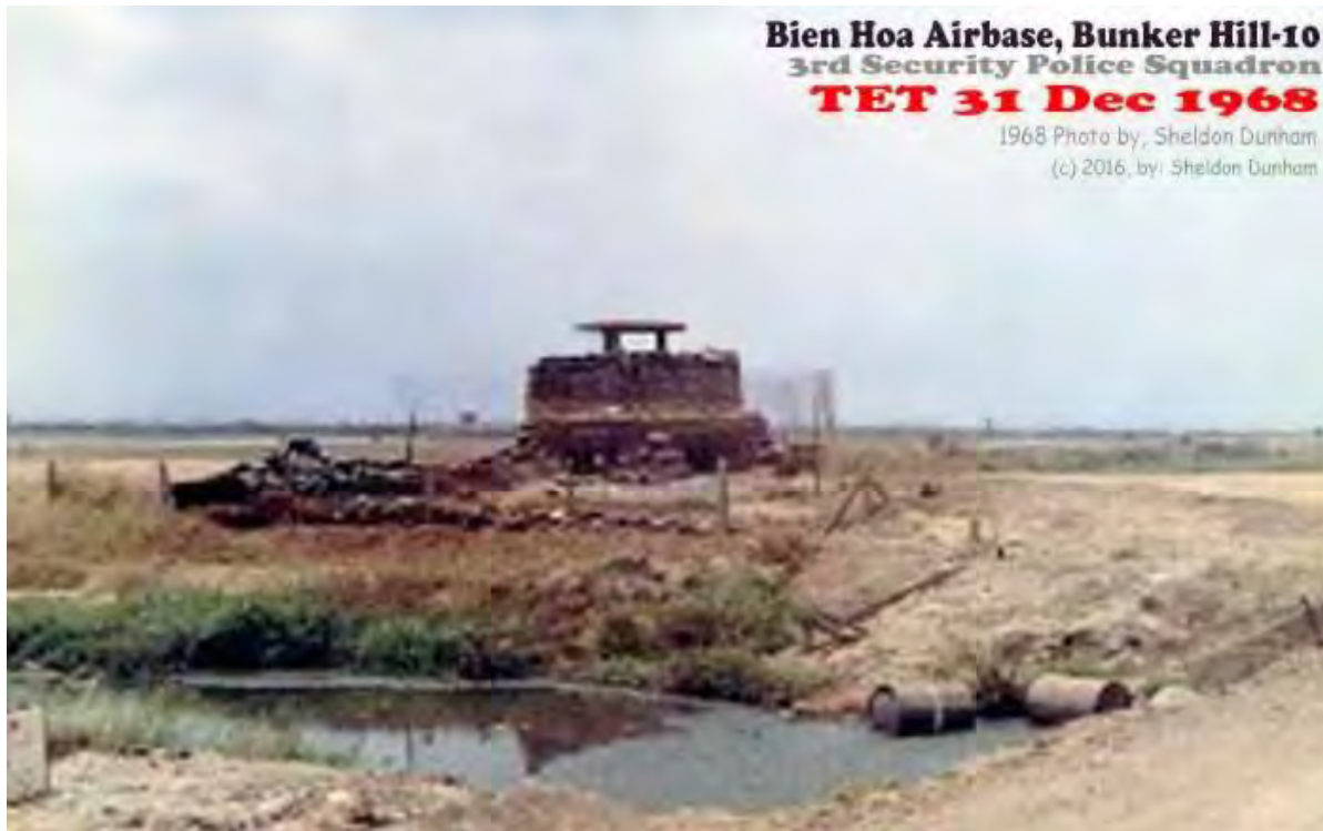
Bunker Hill-10, Bien Hoa Air Base, Tet 1968.
