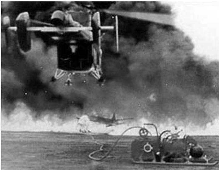
*Firefighters at Phan Rang AB, South Vietnam use an HH-43 to battle a simulated aircraft fire. Source: U.S. Air Force*
