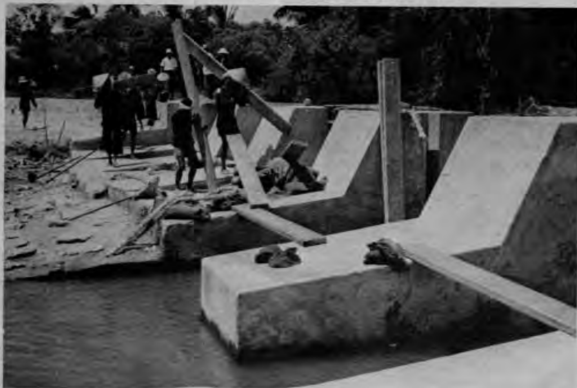
Koreans assist with a dam construction project in Binh Dinh.
