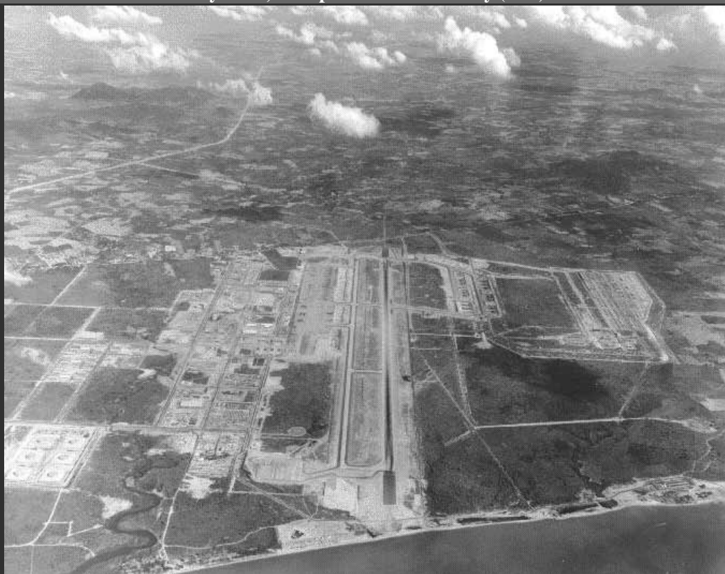
Fly Over, U-Tapao RTAFB Runway (East)
