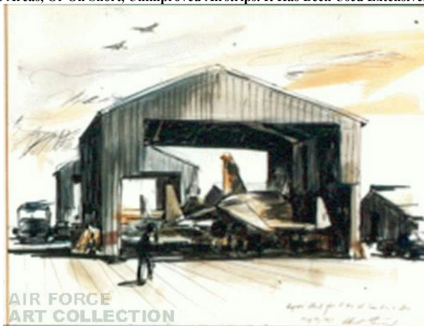
Repair Shed for F-4s at Phu Cat, 1967
