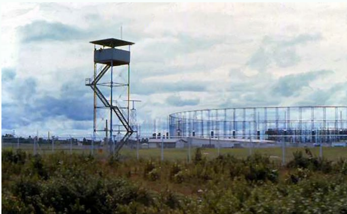
3. Perimeter Tower, with background of Ramasun Station, Thailand, located about 15 kilometers south of Udon RTAFB. Ramasun Station was an Army Security Agency (ASA) station with about 1,000 men from the ASA, USAF Security Service, and USN Security Group. Antenna Array. Photo by unknown.
