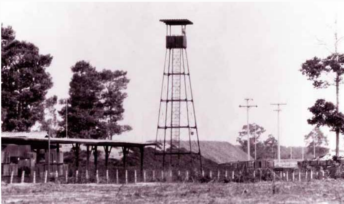
5. Ubon RTAFB. Bomb Dump, Perimeter Texas-Tower, Fox-54. 1970.
