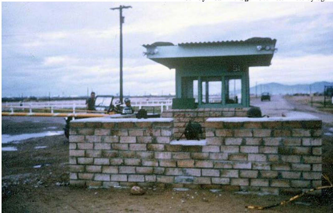
4. Tuy Hòa AB: Main Gate, south. Photo by Sgt DeWhite. 1969-1970.
