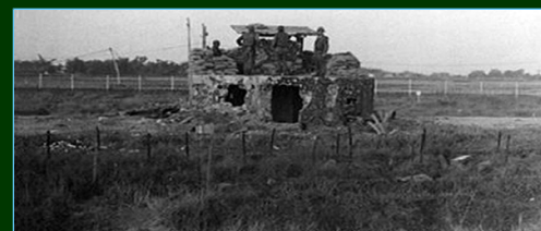
(O51 Bunker as viewed from the rear. Concrete is heavily pock-marked after being overrun by NVA/VC, and then recaptured by Air Force Security Police)
