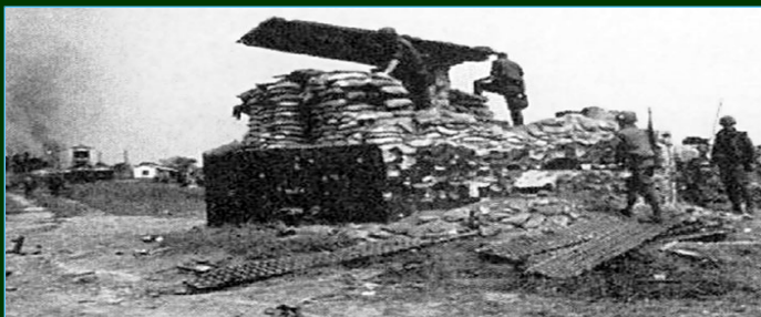
O51 Bunker, 1968, USAF Security Police, after battle for Tân Sơn Nhứt (Viewed almost from the same angle as above)
