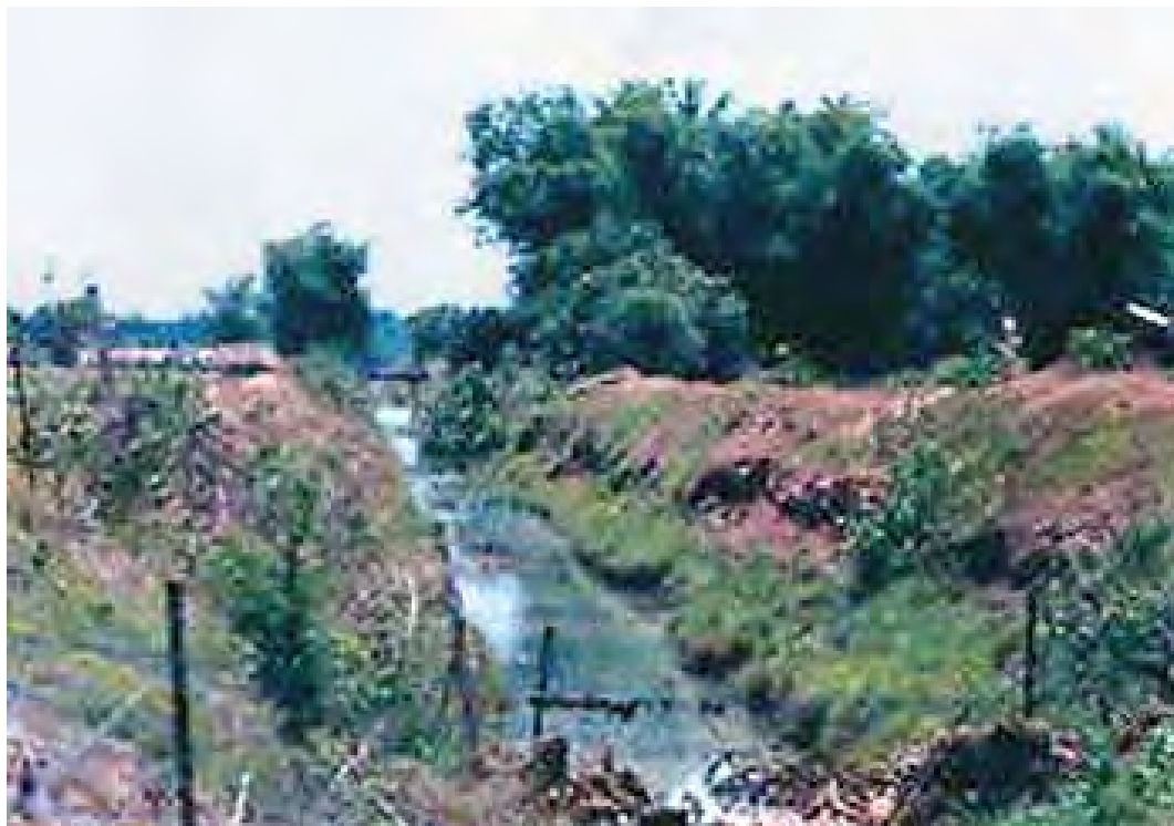
Photo below: Utah Ditch
