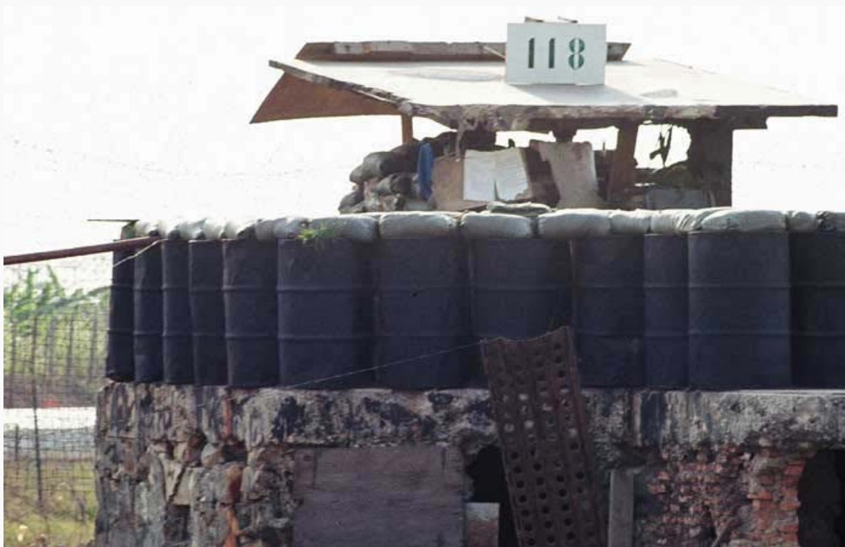
23. Tân Sơn Nhứt AB: Bunker BB7: 051-Bunker, viewed from rear.
