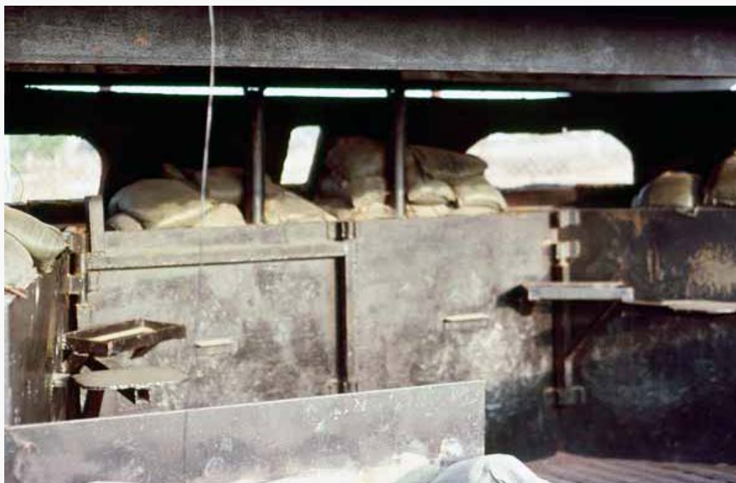
19. Tân Sơn Nhứt AB: Bunker BB7: This is looking inside BB7. They were made of 3/4" steel with a wall like the insided of a house with dirt in the middle. In front of the bunker were sandbags and then 55gal. steel drums. also there was a cyclone fence surrounding it. this was tp prevent mortars hitting the front.
