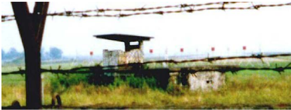
10. Decades later, a revisiting ex-Security Police 'tourist' pestered his tour-guide for permission to stand atop their parked vehicle and raise his camera over the fence for a photo of O-51 Bunker, as it appears today. Standbags have long since melted away, but the blood of four KIA SPs and hundreds of VC and NVA remains a part of that battlefield of Tet 1968. Photo by unknown.
