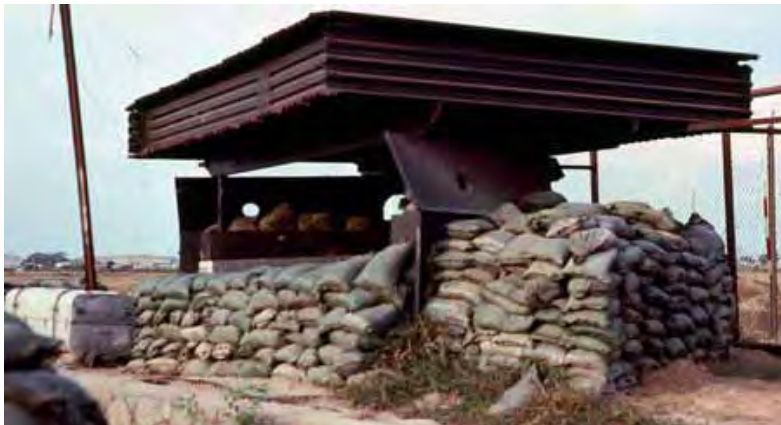
33. Tân Sơn Nhứt AB: Bunker BB7: Right side of bunker. Extra ammo can and cleaning supplies were chained up in a transfer case in the rear of the bunker.
