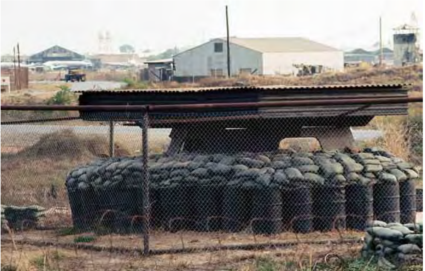
36. Tân Sơn Nhứt AB: Bunker BB7: T-16 showing the fence line to the rear/right with Bravo-Bunker-8 in the rear, the two story one with the pointed roof. Towers in background.
