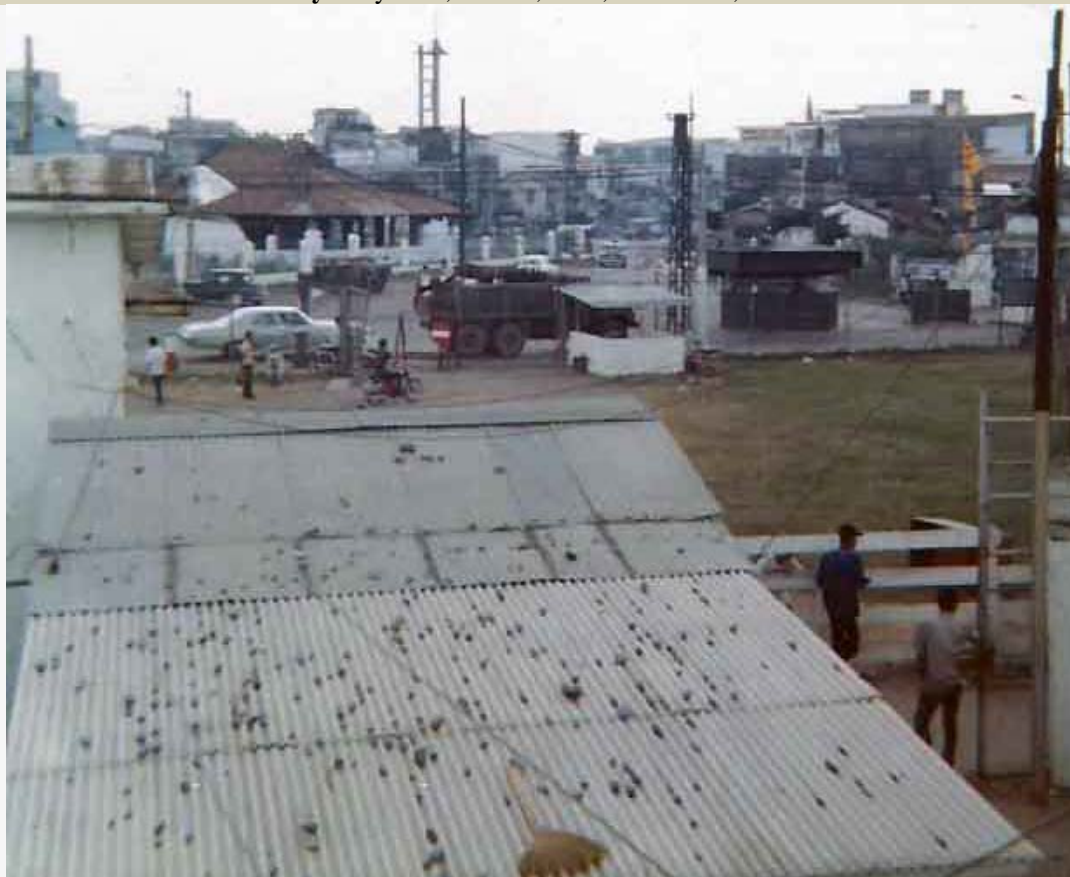
25. Tân Sơn Nhứt AB, Main Gate Tower view. 1972. Photo by Gary Bird, LM 76, TSN, 377th SPS, 1972-1973.
