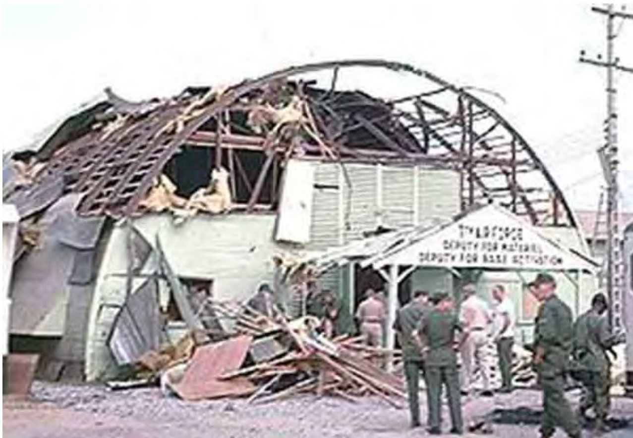
14. Supply headquarters hit by a rocket.
