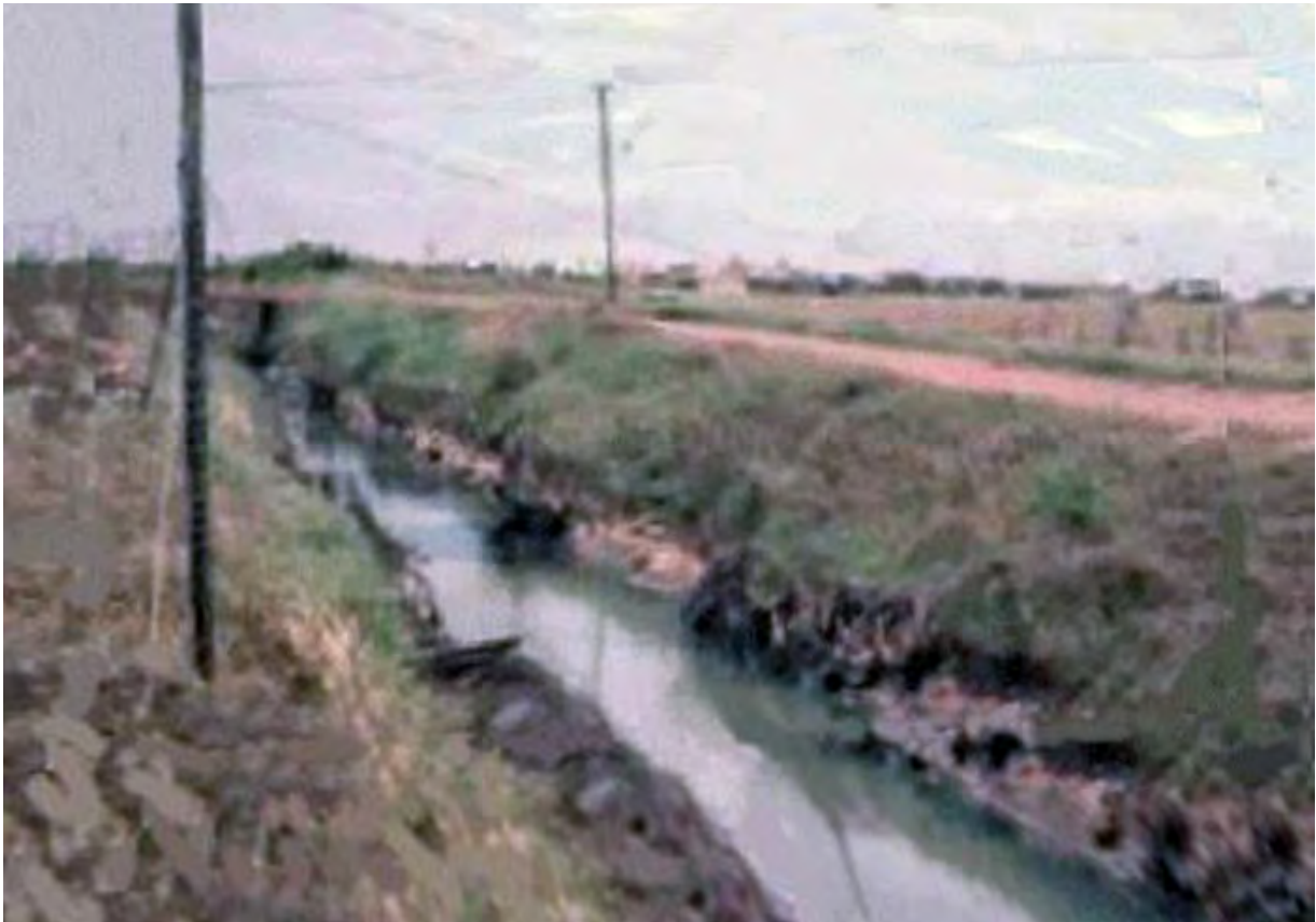
17. Utah Ditch: looking from the fence-line into the base.
