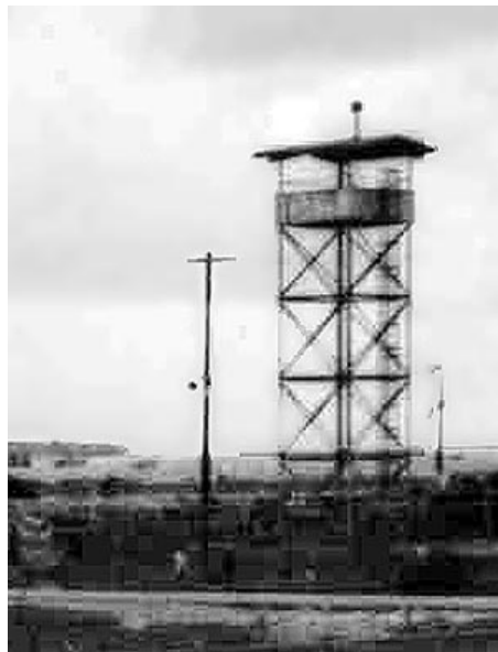
9. Tan My, Loran Station. Tower. Det-1. 1972. Photo by Michael Douglas, 1972.
