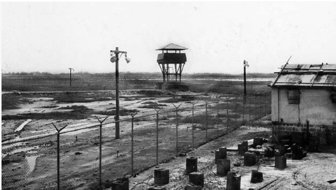
4. Tan My, Loran Station. Perimeter Tower. Det-1. Photo by unknown.
