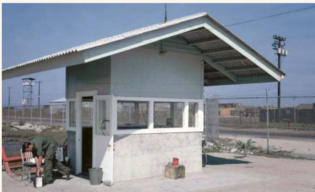
1. Tan My, Loran Station Main Gate. Not only was this our Main Gate, it was also our CSC! All photos were taken in 1971. Note Tower-63 visible beneath gate's eaves (above Airman). Photographer: Jim Burke, LM 466, DN, 366th SPS; DET/TMY, 1970-1971.
