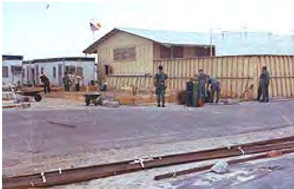
51. Construction of the warehouse.
