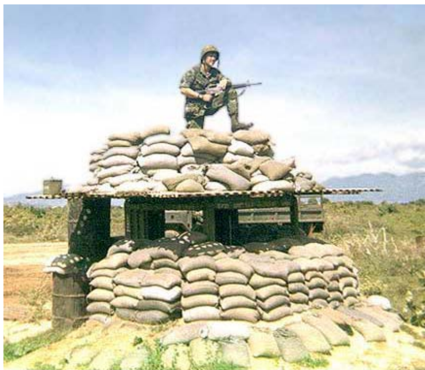
Another Bunker in "Juliet" sector, PhangRang 1970-71
