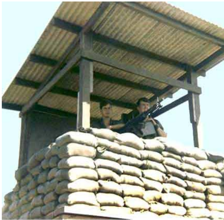
Bunker "Juliet 18" PhanRang perimeter 1970-71.
