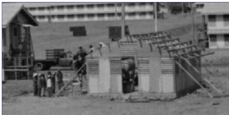
2) Vietnamese civilian workers perform construction.
