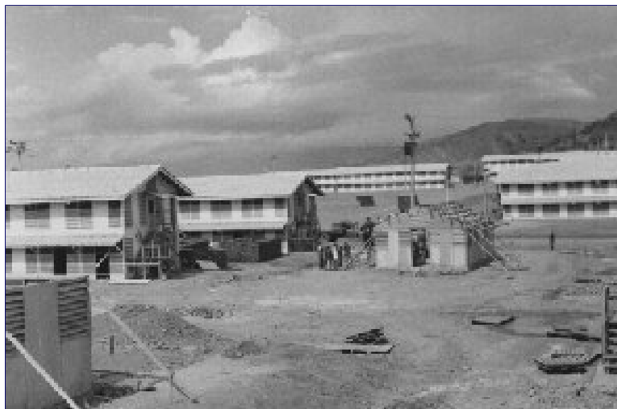
1) New barracks under construction.
