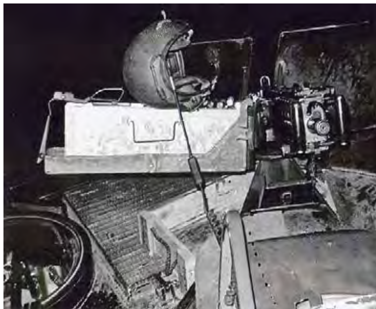
38. Phan Rang AB, V100, M60 with aircraft trigger system.
