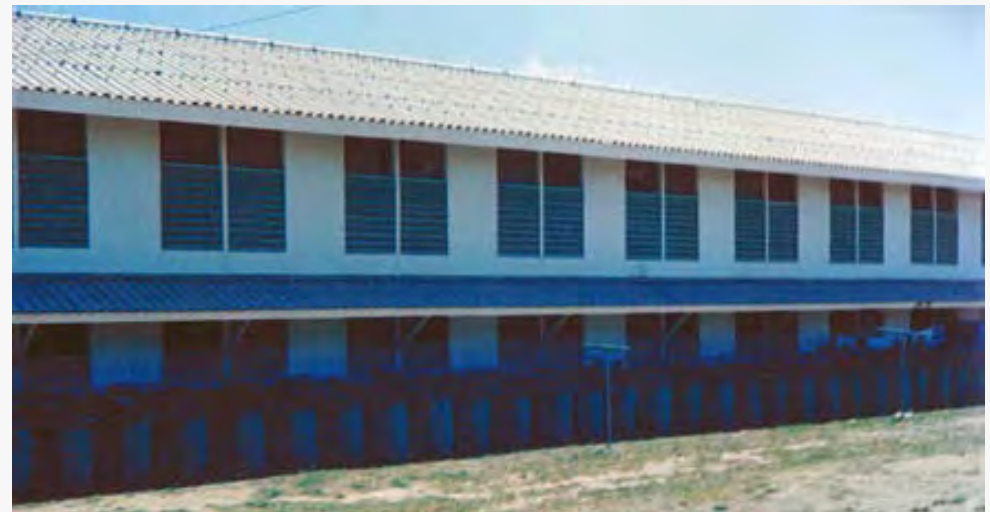
32. Phan Rang AB: 35th SPS Barracks (outside sandbag shrapnel barrier).
