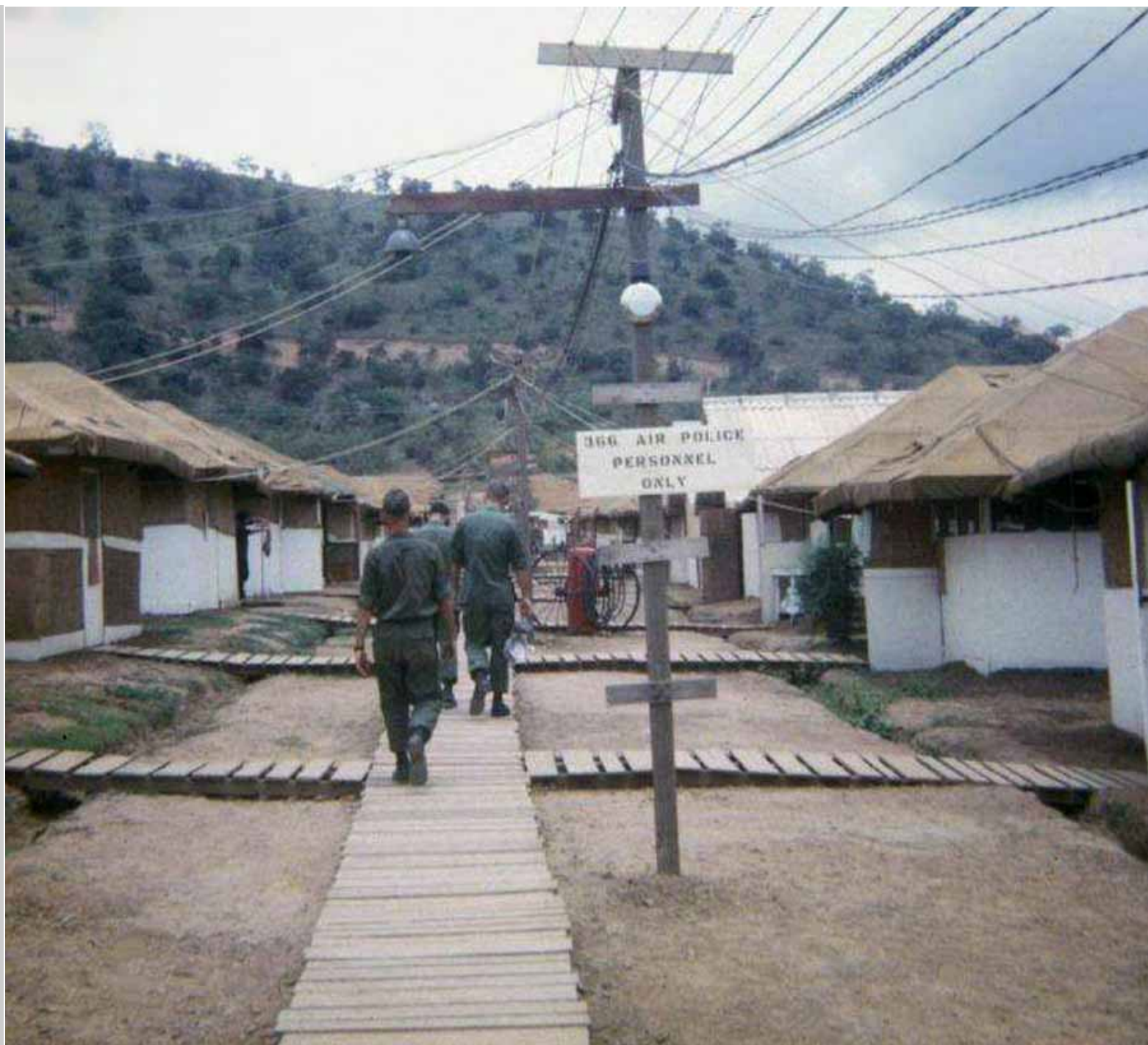
2. Phan Rang AB: Nui Dat Hill, 366th APS: Tent-Huts and wooden plank-walks for monsoon weather, with Nui Dat Hill in background.
