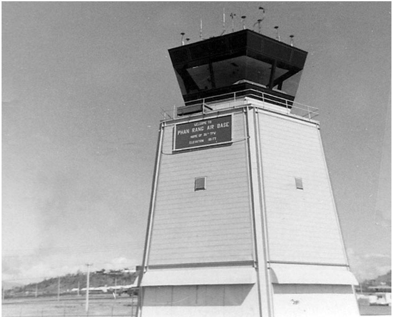
7. Phan Rang AB: Control Tower. Photo by Van Digby, 1967-1968.
