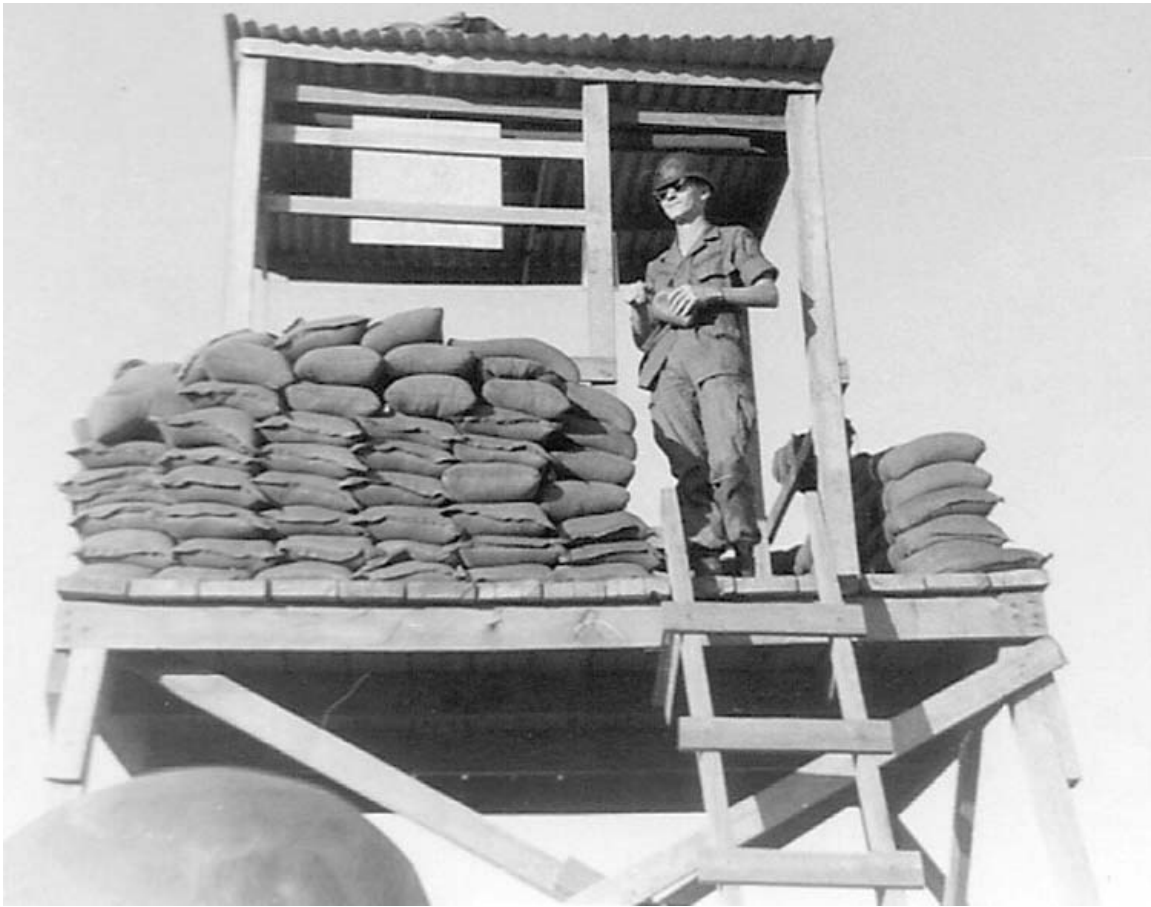
16. Phan Rang AB: Bunker Tower OP-4, A2C Hatley. Photo by Van Digby, 1967-1968.
