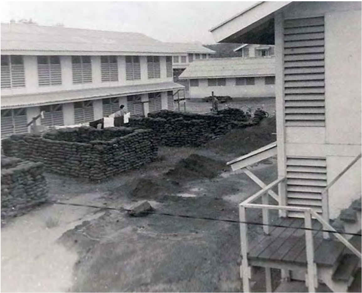
18. Phan Rang AB: Barracks Area under construction. Photo by Van Digby, 1968.
