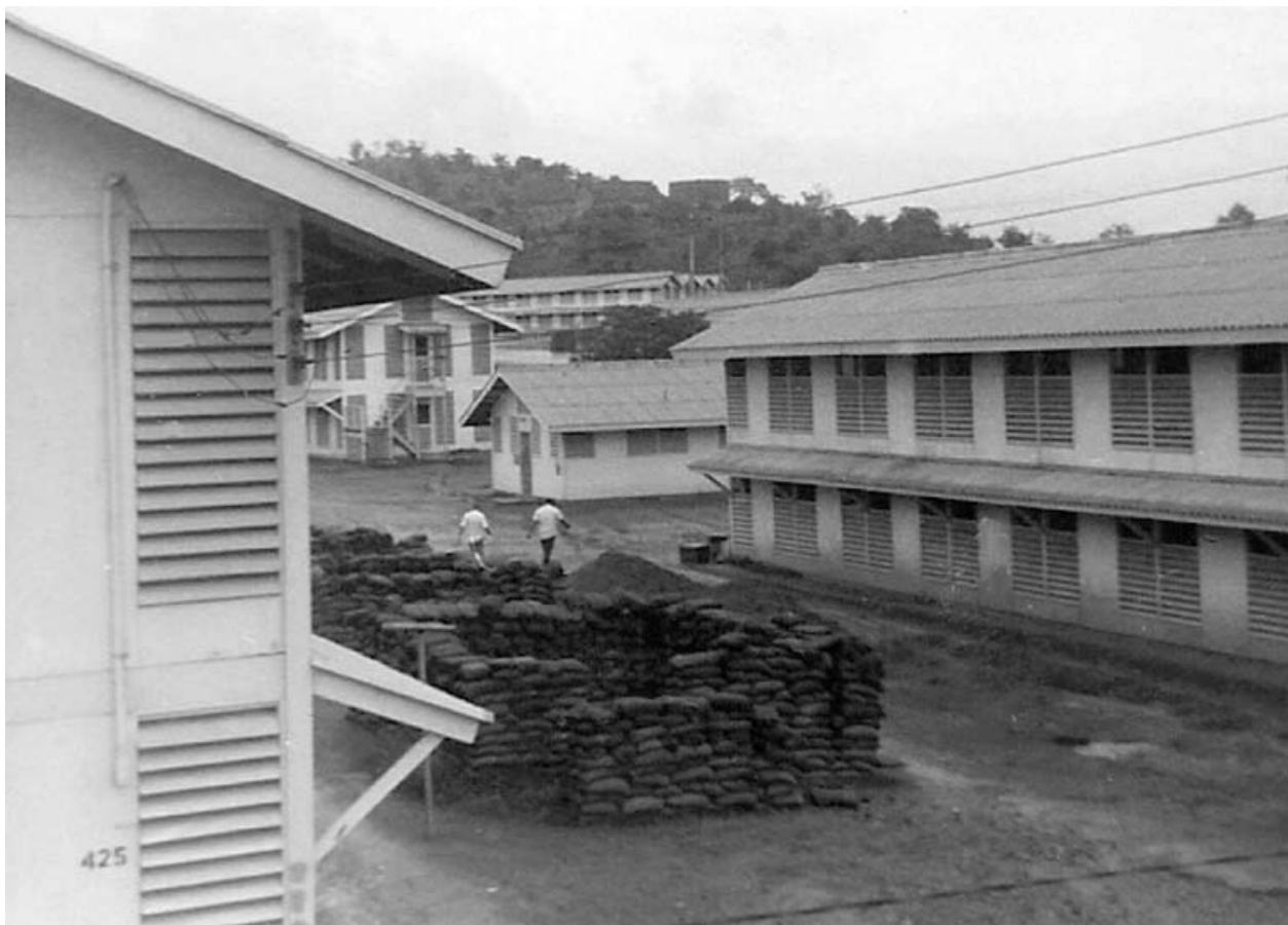
17. Phan Rang Barracks Area under construction. Photo by Van Digby, 1968.
