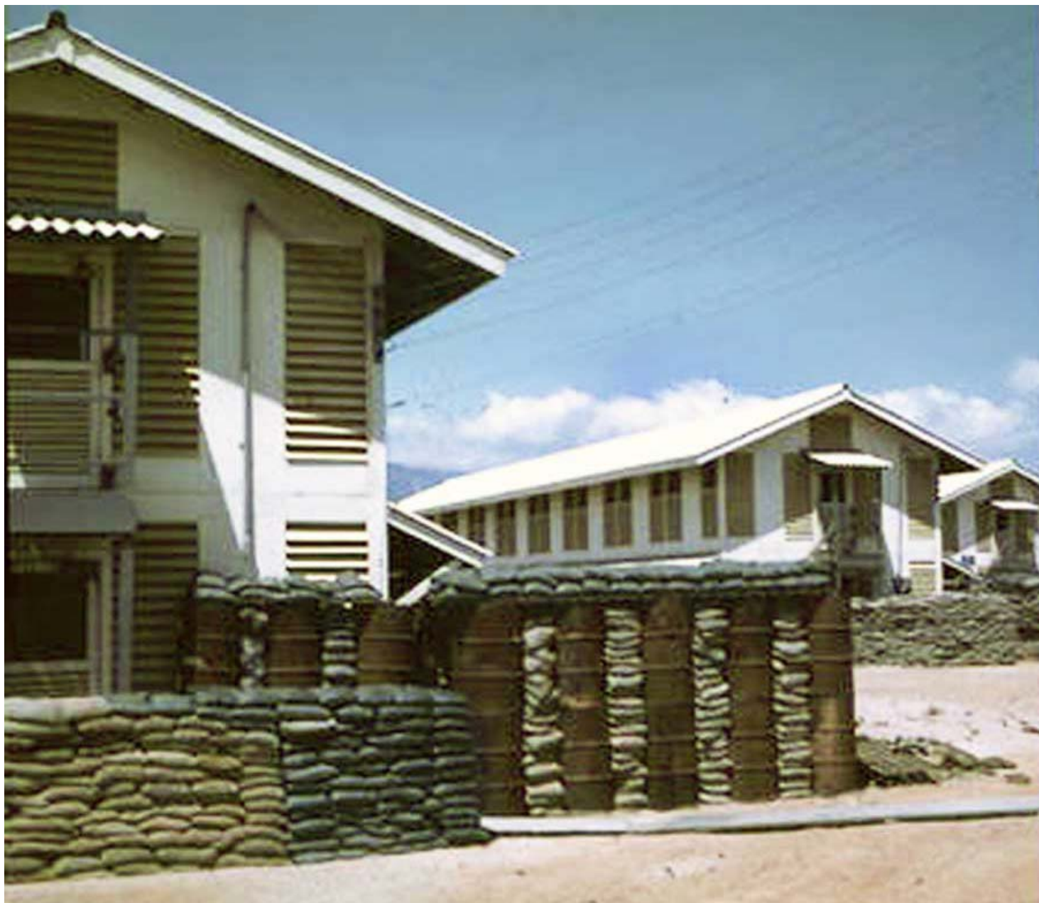
11. Nui Dat: 35th SPS. With barracks construction, followed sandbag and bunkers details. I wonder what the barrels had contained? Photo by Stan Reeves, ND 1967.
