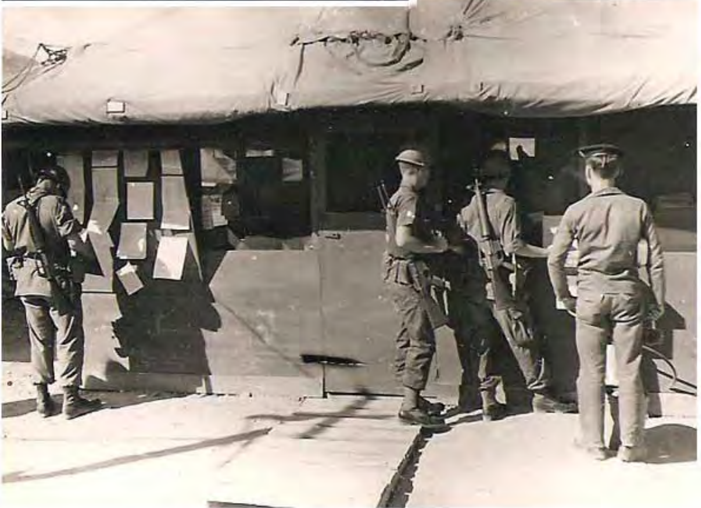
26. Top-Left: Main Entrance.
