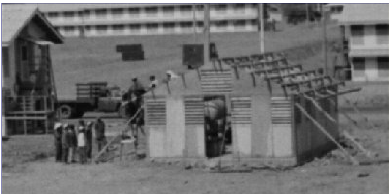
2) Vietnamese civilian workers perform construction.
