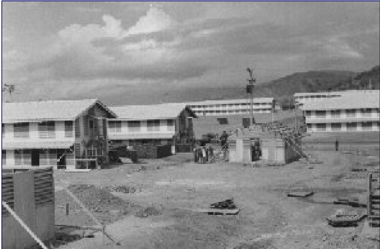
1) New barracks under construction.
