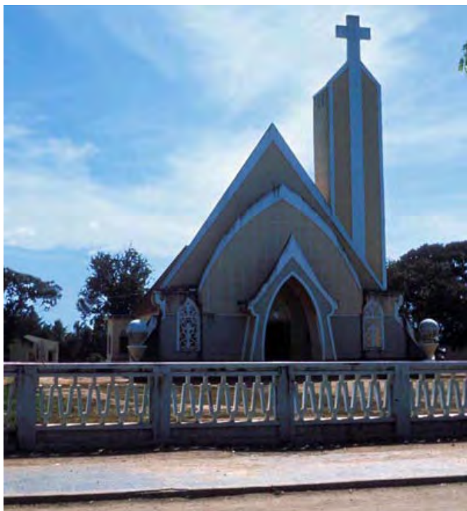
49. Phan Rang: Christian Church across the bridge.
