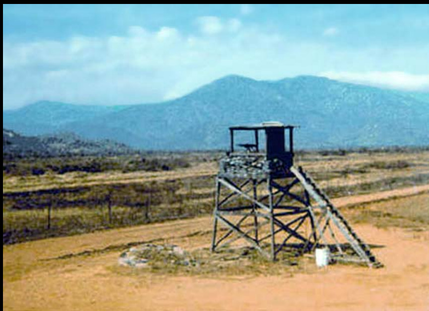
Photo below: Sgt Gover getting ready for overnight Juliet tower posting on the East perimeter of Phan Rang AB.
