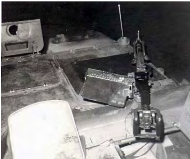
22. Phan Rang AB, V100, M60 with aircraft trigger system.
