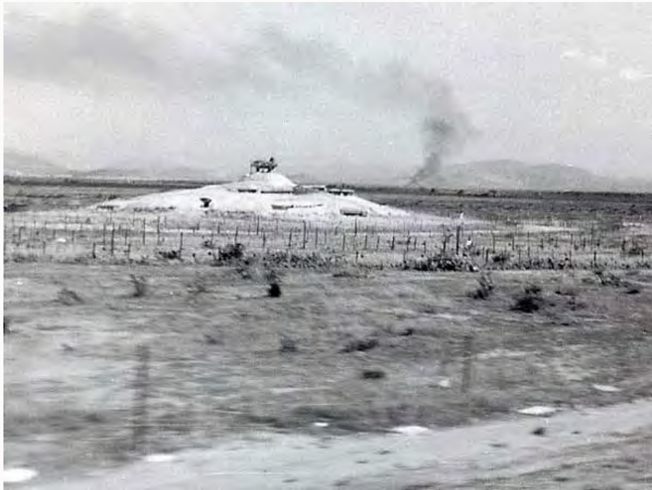
13. Phan Rang AB: Hwy 82, Road to the Beach: Bunker and Mine Field.
