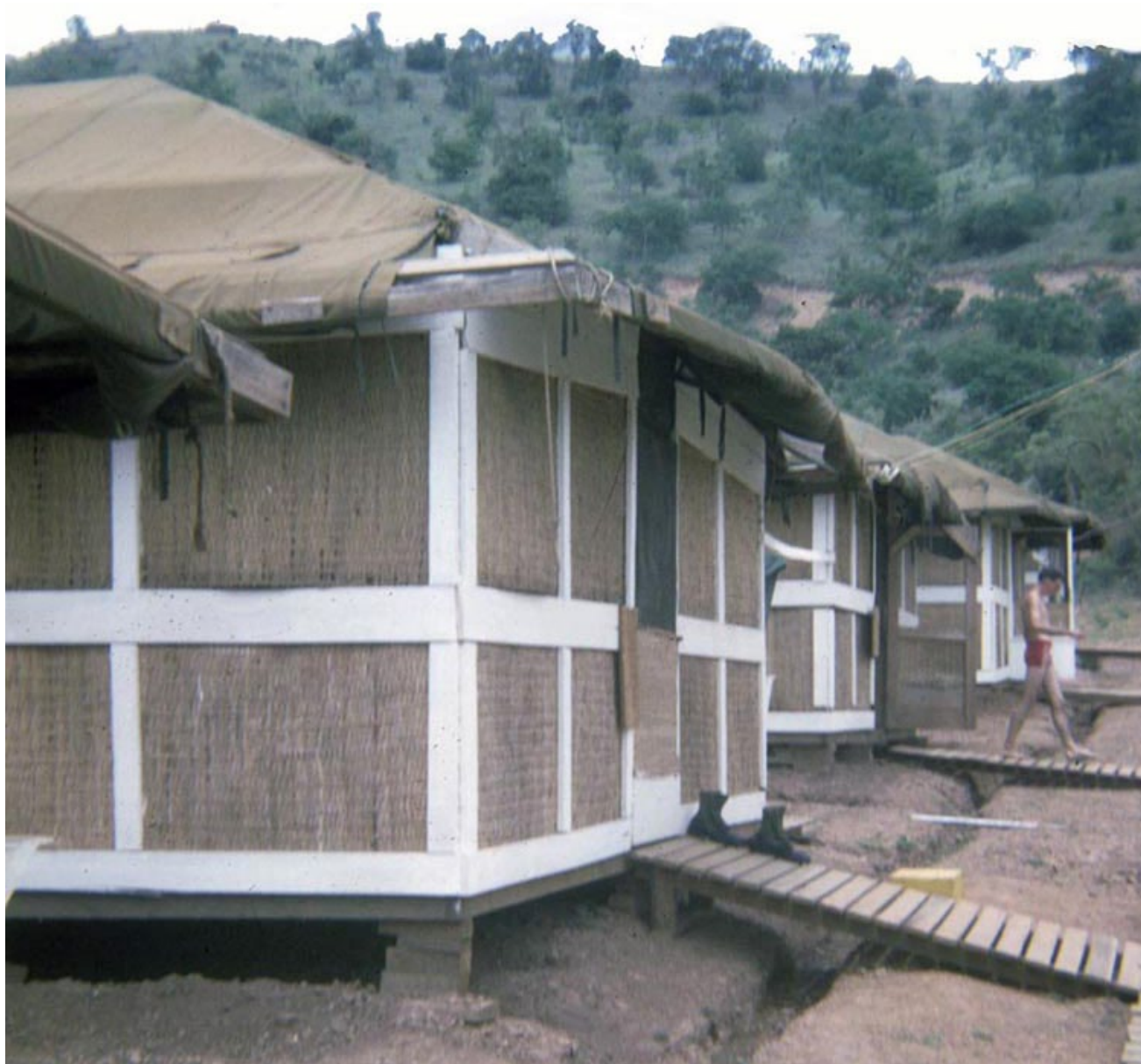
20. Phan Rang AB: 1966: New tent-huts, with wooden walkways and storm drains.
