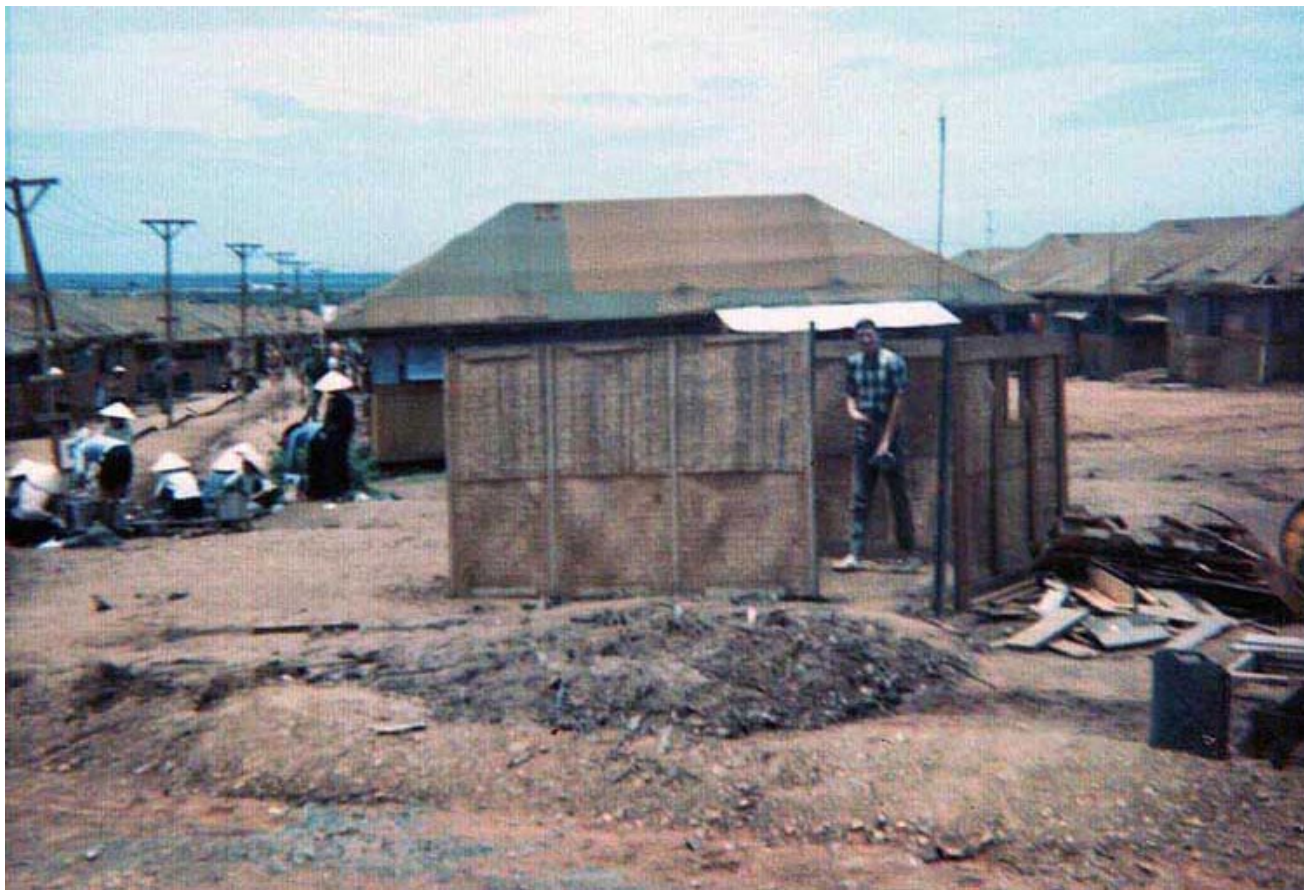
24. Phan Rang AB: Piss Tube with courtesy-walls (early on, there were no walls). HEY!!! Is nothing scared anymore?
