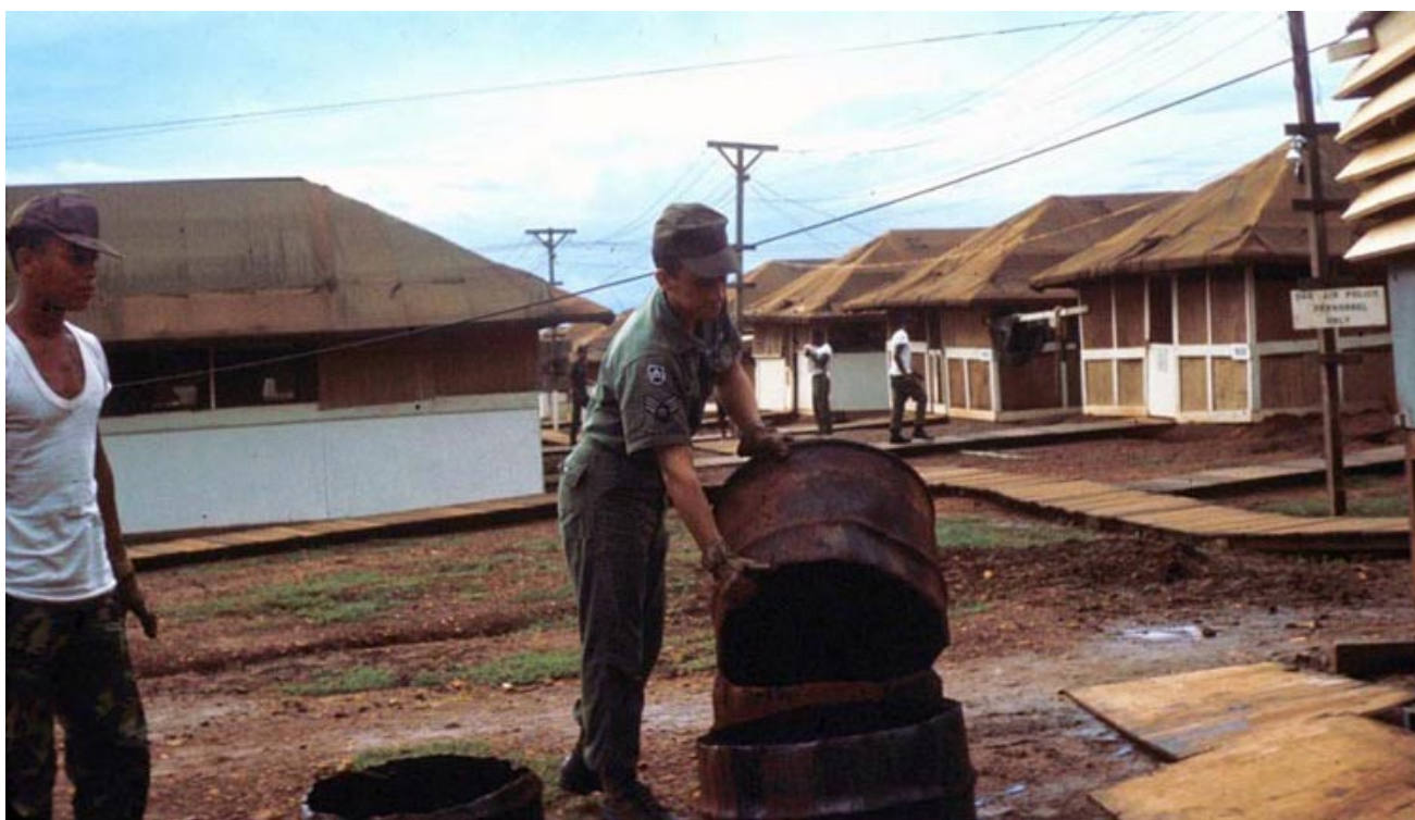
35. Six Hole (8 holes?) Outhouse Stuff Burning Detail.
