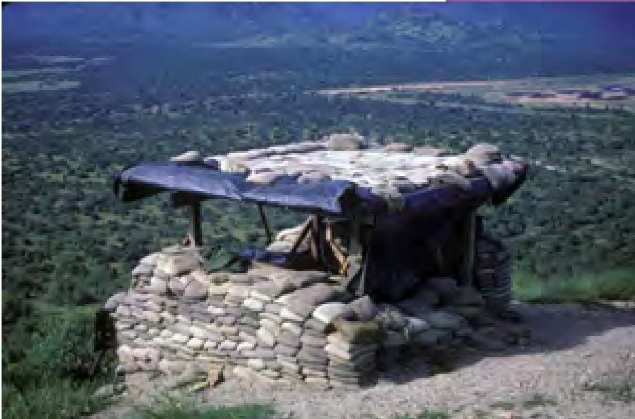
3. Phan Rang AB (below): OP-2, a bunker fortified with PSP and sandbags, armed with an 50.cal machinegun, overlooks the valley below and the bomb dump (right).
