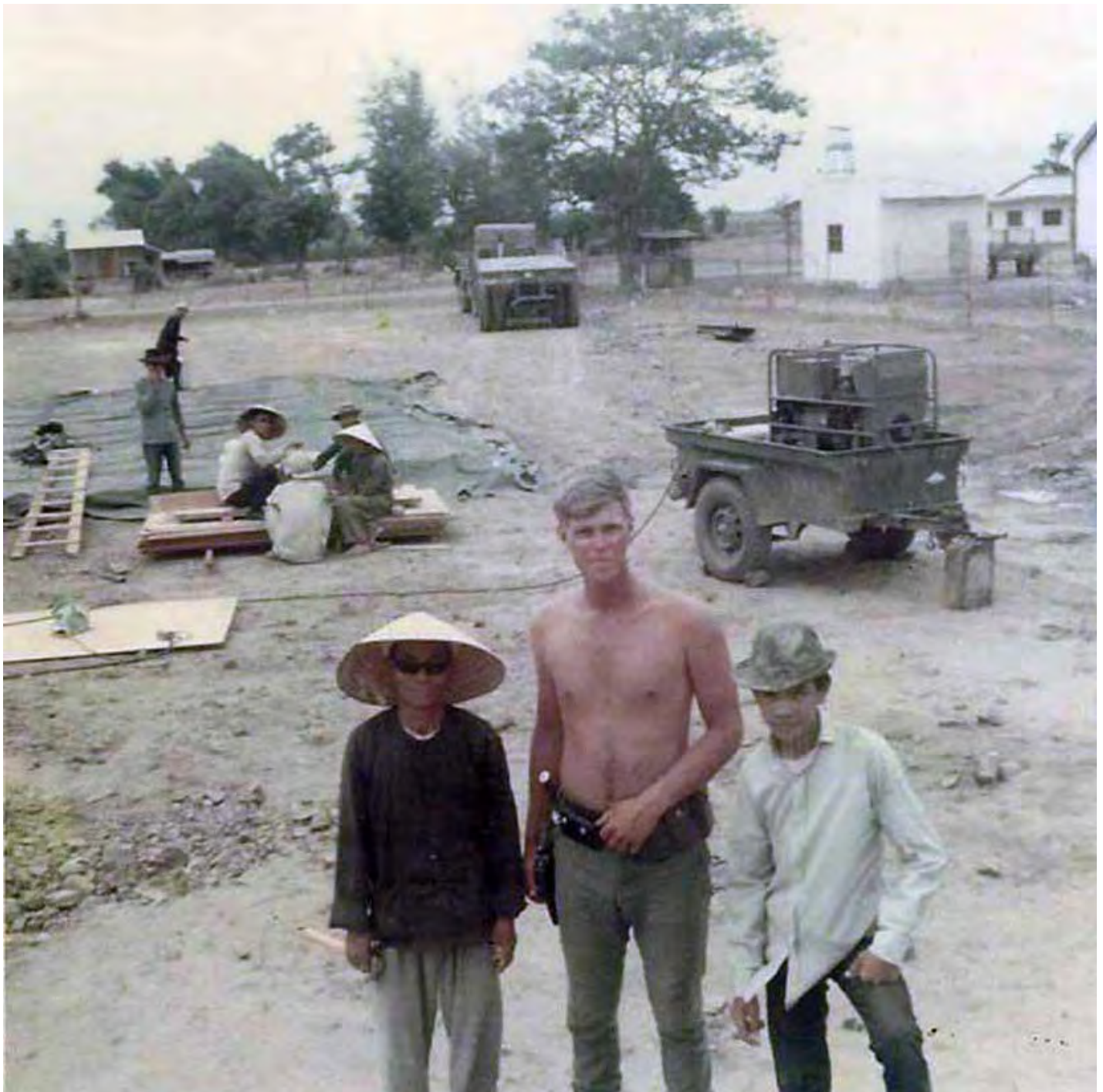
9. Phan Rang AB: Waterpoint Bunker, Outside of Base. Vietnames Workers. Photo by Dana Anthony, 1968-1969.
